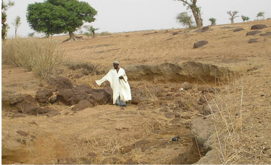
Gullies due to water erosion
